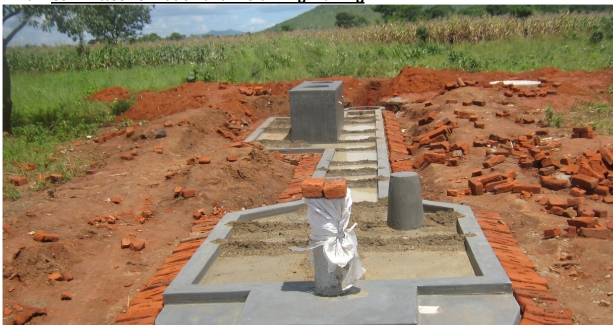
Chimuti water point in Mchinji, T/A Zulu under construction: 2009
